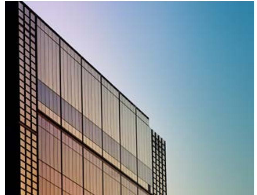
Baillie Gifford's new Haymarket office, set to become SAINTS' sixth Edinburgh home in 2024
